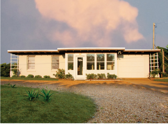
Foundation office at 13 Skyline Road
